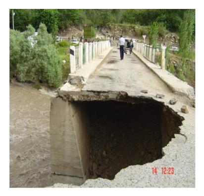
Figure 10. Damaged bridge in Varzob Distrikt
